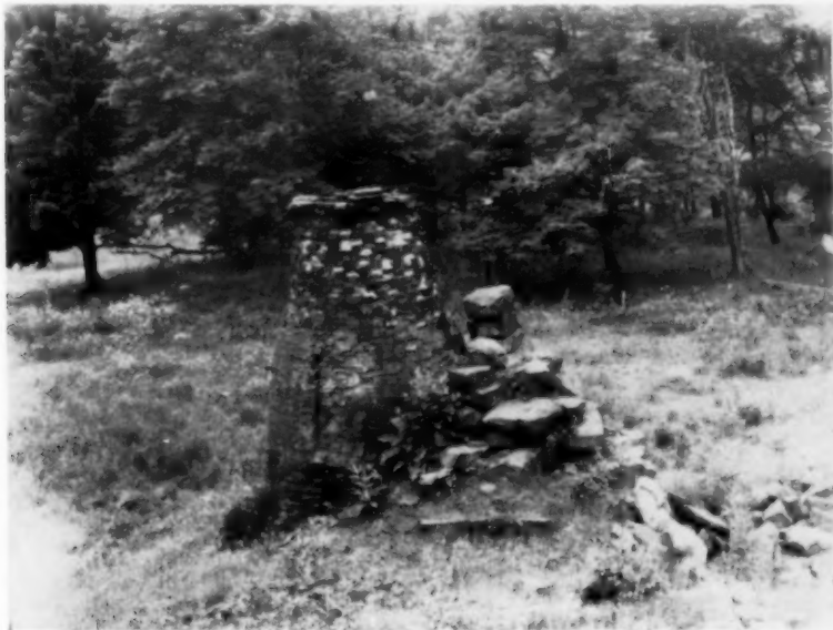
Shippen Furnace: Example of badly ruined remains.
